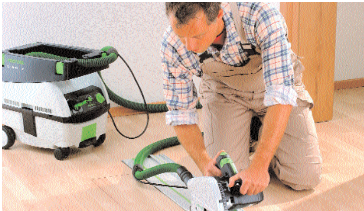
Using the TS 55 to saw timber floors: clean and quick.
